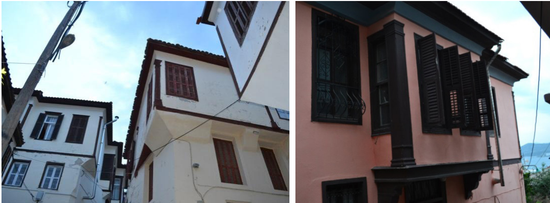
Different types of bay windows, methods for straightening the top floor plans (Source: Velika Ivkovska, 2014)
