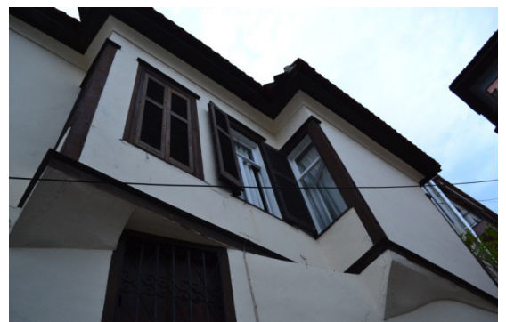
Types of bay windows, and consoles as methods for straightening the top floor plans (Source: Velika Ivkowska, 2014)
