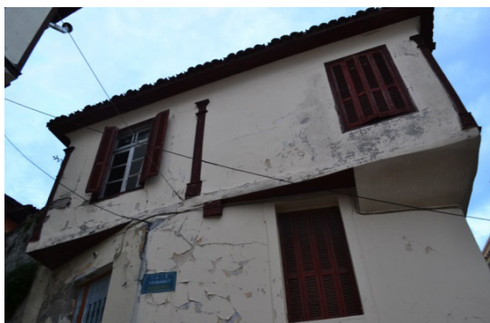
Types of bay windows, and consoles as methods for straightening the top floor plans (Source: Velika Ivkowska, 2014)
